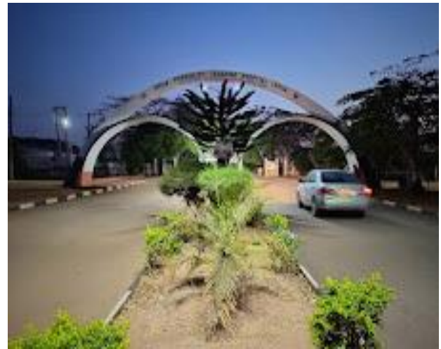
Figure 1 Entrance gate to ISTH Irrua
